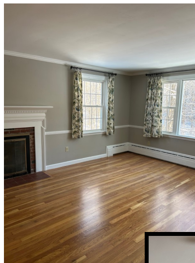
Left is a photo of the refinished wood floors and the ceiling repair and fresh paint in the living room of the parsonage. Nice work Property Committee!
